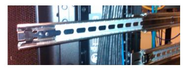
10. Carefully lift the chassis and align slide-chassis members with the slide-cabinet member black plastic alignment pins.
